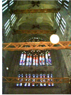
Figure 2: Ad hoc measures preventing the Beauvais cathedral from collapsing.
