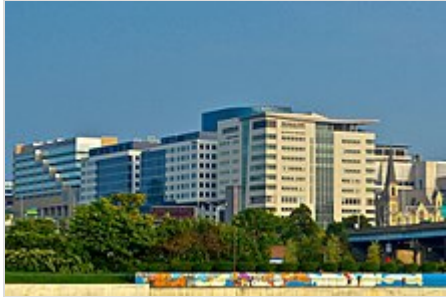
A collection of Spectrum Health facilities and affiliates on the Medical Mile .
